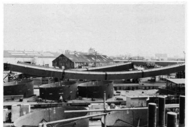
Fig.7 Temporary assembly of the upper chord member
